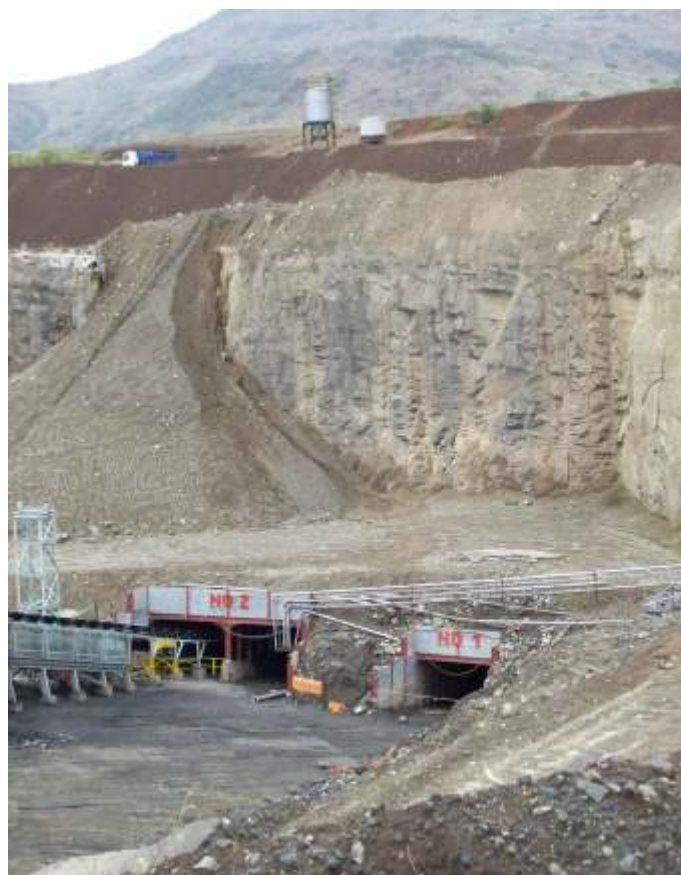
View of silo and 35m drop to mine tunnel
